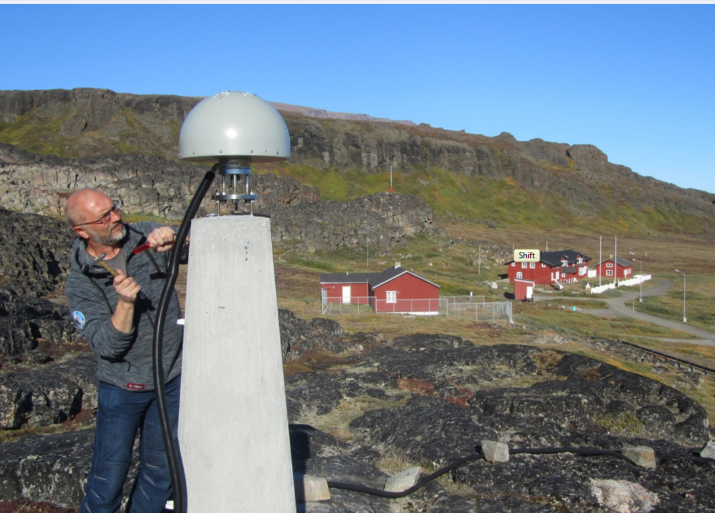
Bjørn-Ove Husøy removes a small amount of concrete from the top of the pillar to make room for the repaired cable. Photo by Lars William Pedersen.
